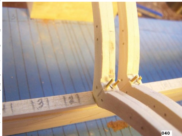
Frames attached to the keel
